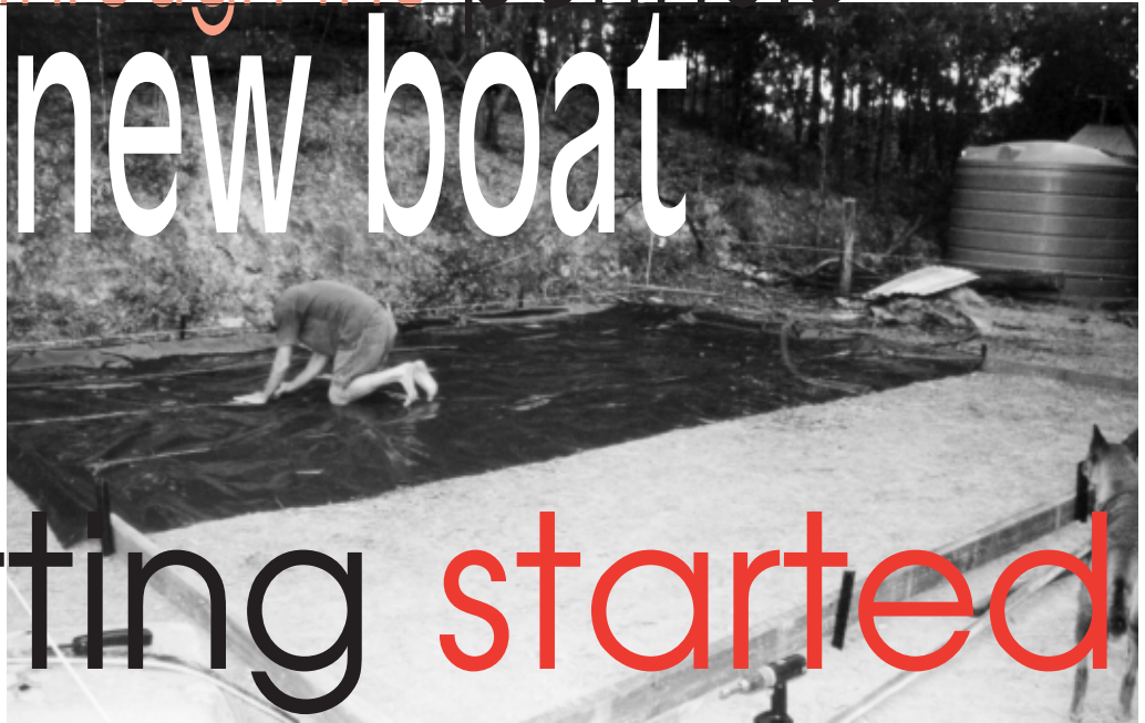
GETTING the plastic down prior to concreting
